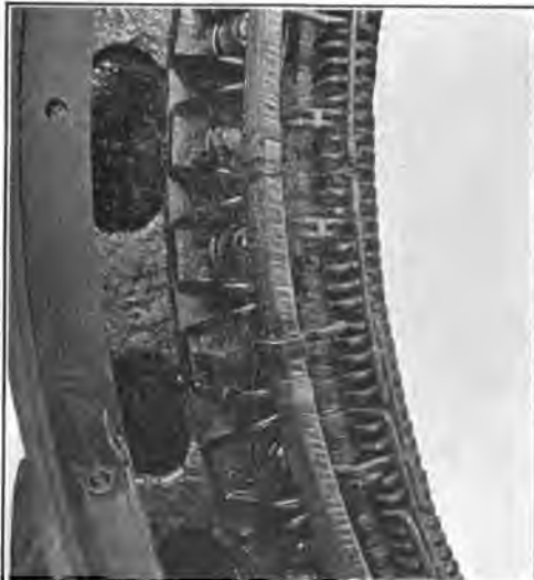
FIG. 63.—U. S. S. New Mexico : Method of Securing Stator End Winding
